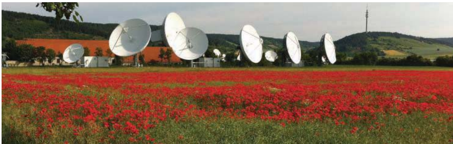
Intelsat's teleports in Fuchsstadt, Germany. Photo courtesy of Intelsat.
